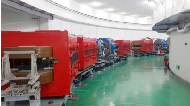
Figure 10: The dipoles and quadrupoles installed in the tunnel.
