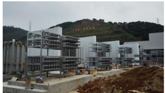
Figure 13: The choke and capacity bank for WHITE power supply.
