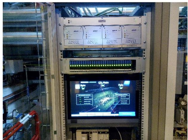
Figure 2: 24V DC power supply & distribution, Touch panel and PLC.
