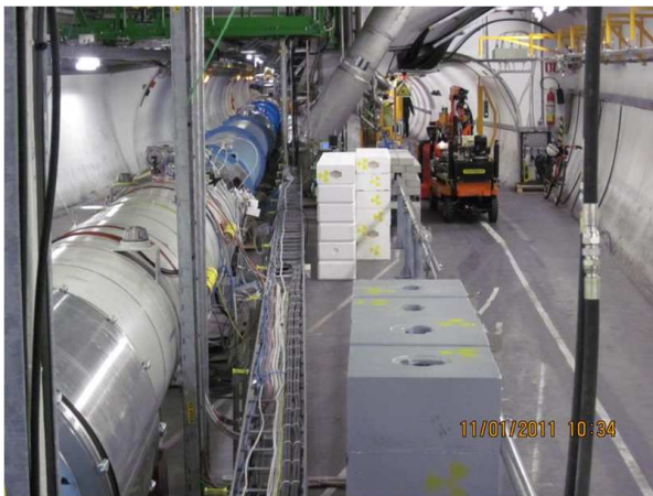
Figure 7: Shielding blocks installed in UJ22. On the right the incoming TI 2 line, upstream view.
