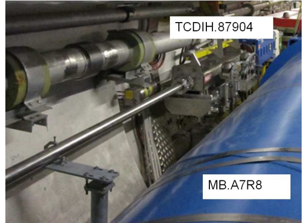
Figure 8: Limited space for shielding at TCDIH.87904.
