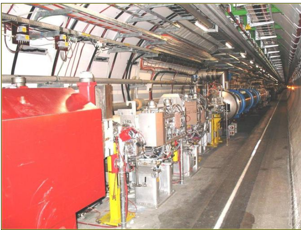
Figure 4: Beam instrumentation, collimators and other equipment presently installed in between the TAN (red object on the left) and the D2 separation dipole (blue cryostat on the right) in the ATLAS matching section.
