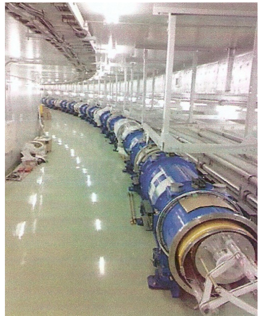
Figure 4: Installed superconducting magnet system in the J-PARC neutrino beam line.
