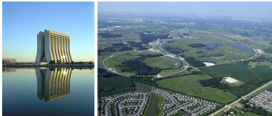
Figure 4.1: Wilson Hall, and the Tevatron
