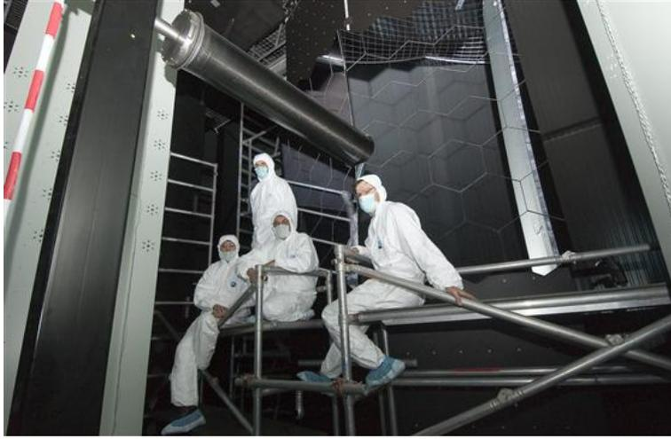
**Figure 2.26:** The RICH2 subdetector under construction, with the spherical mirrors and beam-pipe visible.
