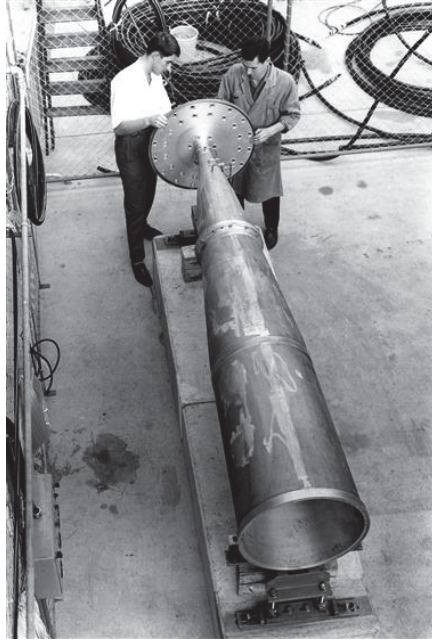
Fig. 3.20. Inner conductor of magnetic horn for neutrino beam.
