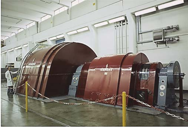
Fig. 3.16. The 2nd generation PS main magnet power supply with the motor in the foreground.
