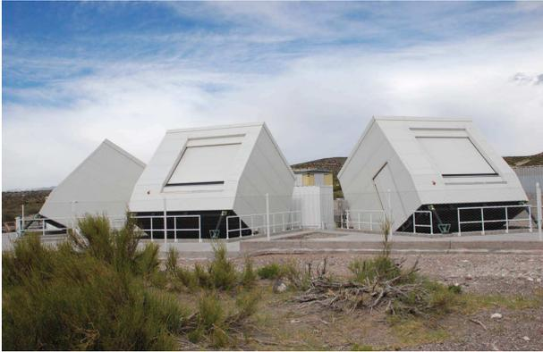
Figure 3: Photograph of HEAT in tilted mode with closed shutters.
