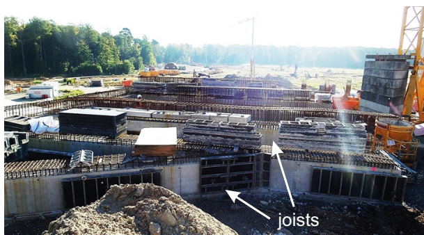
Figure 4: The complete table construction has a piled foundation consisting of 89 pillars. The table itself is supported by reinforced concrete joist as shown in the picture taken during construction.
