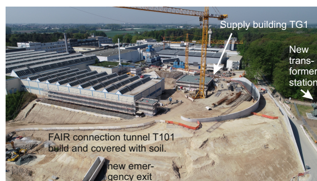
Figure 7: Photo of GAF construction site taken 22th April 2018 by M. Konradt. (GPS: N 49.932879 E 8.682875). The photo is taken from above the FAIR construction site. Clearly visible the new emergency exit. The opening in the existing building and the part of tunnel T101 which have been build are already covered with soil. Most of the table construction on top of the building is covered too. Visible to the right is part of one transformer of FAIR's power station north which is already used to supply GSI's pulsed power grid which feeds the upgraded main power supply of SIS18.
