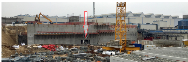
Figure 6: WTK construction works for enhanced transfer channel shielding and the interface of the pLINAC building. The arrow indicates the window for the later pLINAC beam line.
