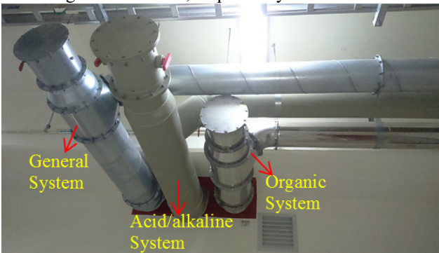
Figure 3: Typical ducts layout of three laboratory exhaust gas treatment systems in a laboratory in the TPS.
