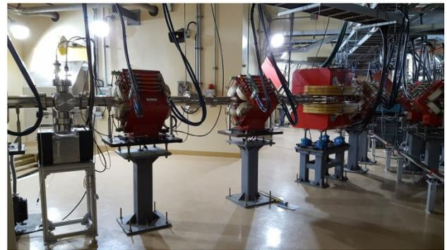
Figure 4: Installed proton beam transport system from AC magnet (right) to the vacuum box (left).
