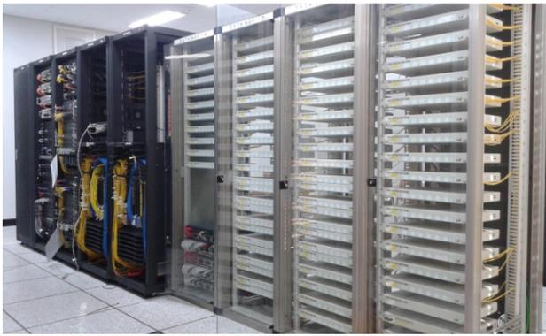
Figure 4: Network core switches and FDFs.
