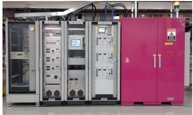
Figure 8: Modulator and its control system.
