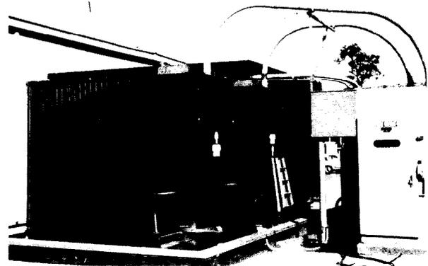
FIG. 4--3.4 MW and 5.0 MW power supply installation. Left to right: shelter, transformers, vacuum switch.
