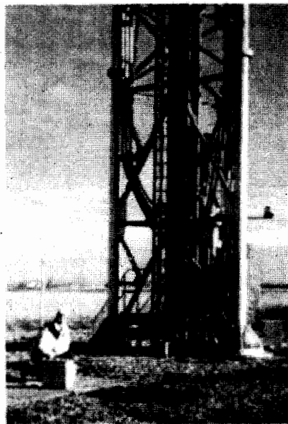
Figure 14 : Base of Erie tower.
