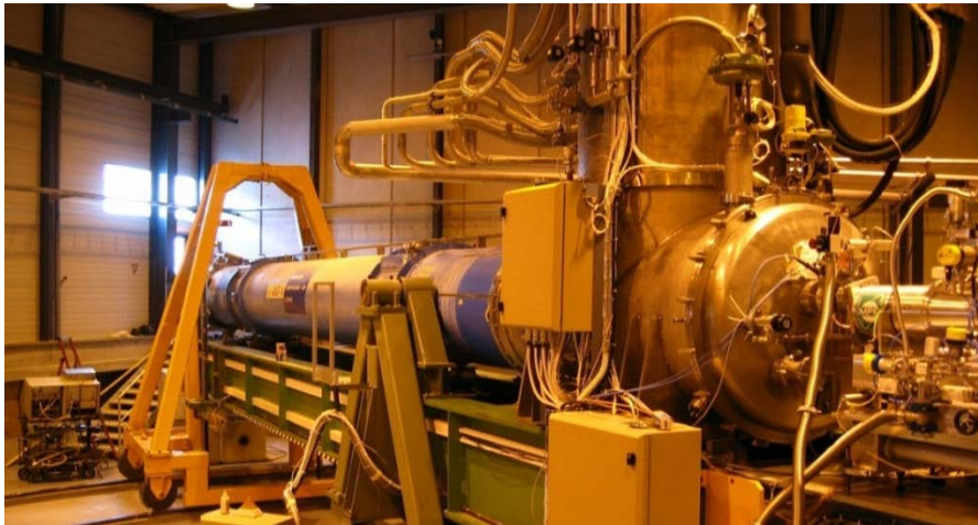
Figure 2.13 View of the window, through which the sun filming is possible twice per year.
