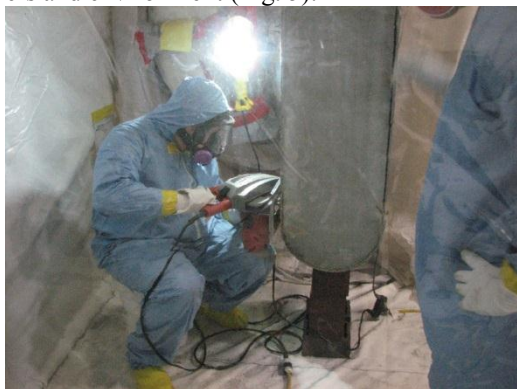
Figure 5: Cryomodule Repair under RWP.
