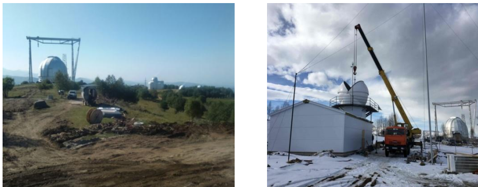
Fig11. Construction of the complex. Left: September 2017. Right: December 2017.
