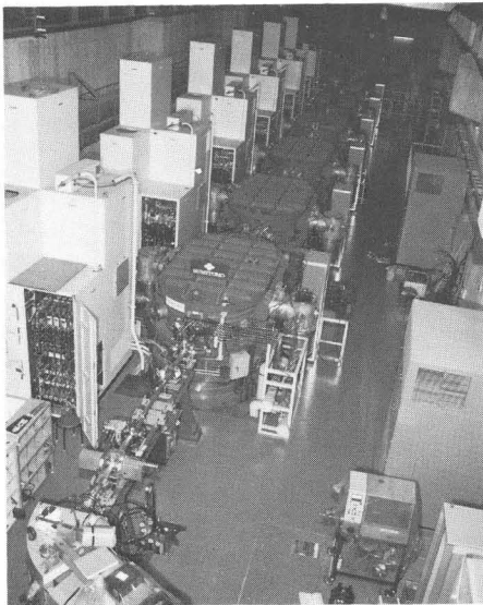
Fig.2. RILAC seen from upstream side.
