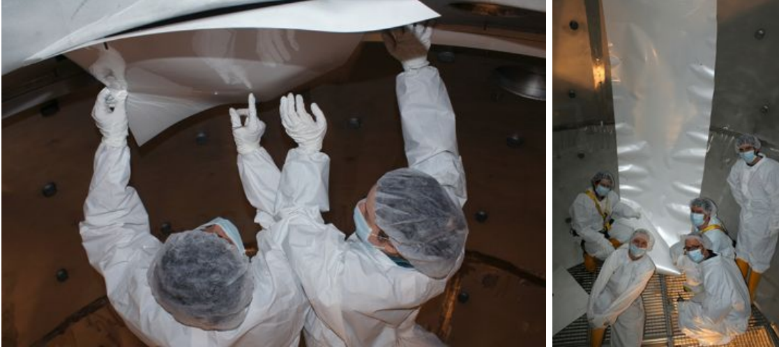
Figure 5.16: Installation of the Lumirror reflector in the DarkSide-50 neutron veto. The Lumirror was held in place by a series of studs welded to the interior wall of the sphere and some Teflon nuts and washers. A similar procedure will be used for the SABRE veto detector.
