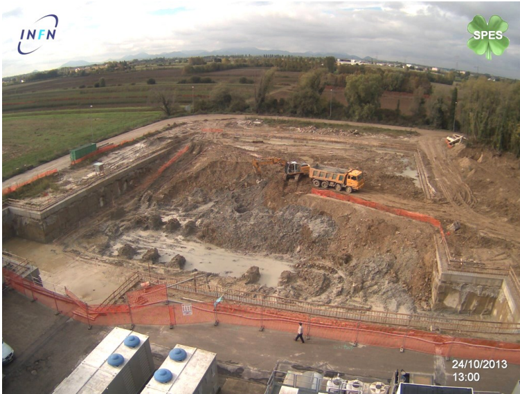
Fig. 2. The SPES construction site.
