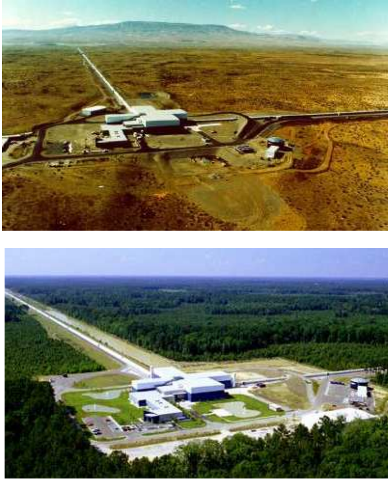
Figure 2.2: On the top: the LIGO (Laser Interferometer Gravitational-wave Observatory) of Hanford, WA. The interferometer is an L-shaped vacuum system which houses 2 co-located detectors (LHO1, 4 Km of arm-lengths and LHO2, 2 Km of arm-lengths) which share the same vacuum system but have different test masses at the extremes. On the bottom: the LIGO facility at Livingston, LA (4 Km of arm-lengths). (Photos: courtesy of the LIGO Laboratory).
