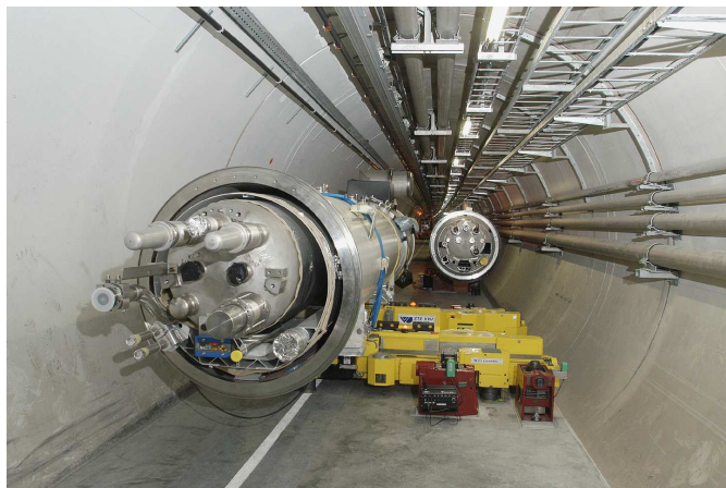
Figure 2.3: Picture of a superconducting magnet being installed in the LHC tunnel, the two channels for the proton beams are clearly visible. LHC will use about 1 200 dipole magnets 14.2 m long which will reach a field strength of 8.3 Tesla.
