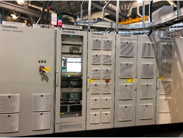
Figure 3: Booster solid-state amplifier installed at the CLS.
