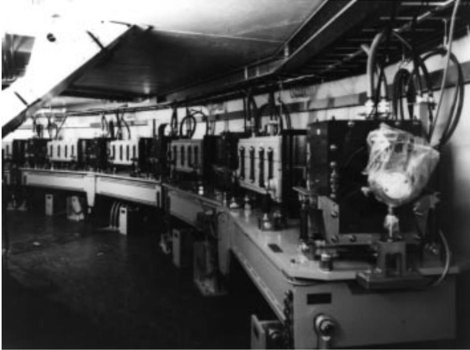
Figure 9. ALS strut supports. Photo courtesy of Lawrence Berkeley Laboratory, University of California.
